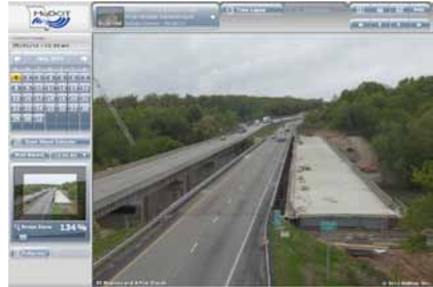
Rather than tie up traffic for weeks by building the new bridge piece by piece at the site of the existing bridge, the general contractor built the new bridge next to the old bridge.
