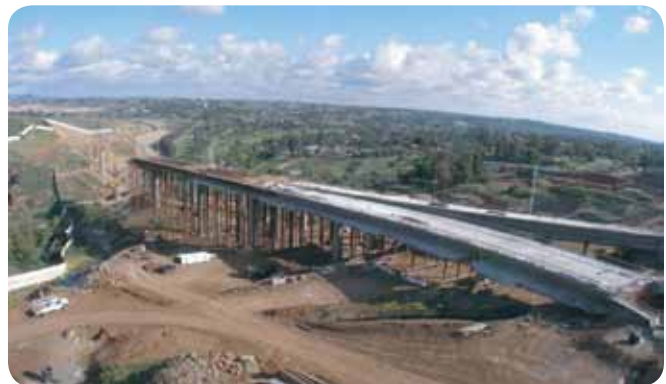
Sweetwater River Bridge
