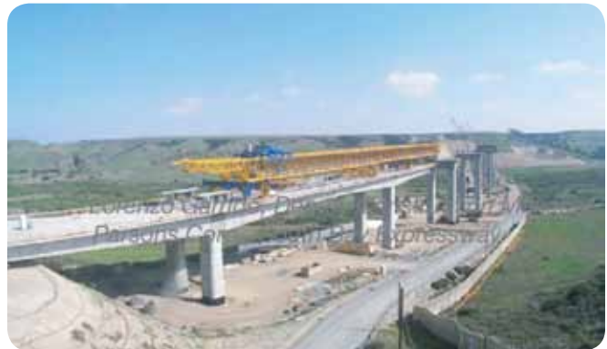
Otay River Bridge
